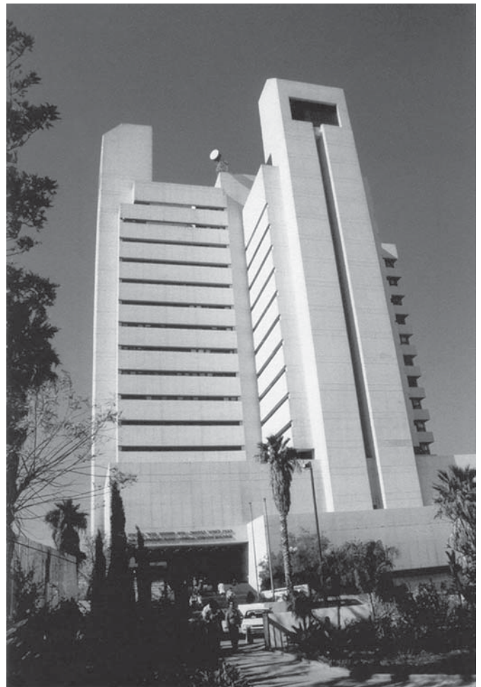
Fig. 3. The Rappaport Family Building for the Medical Sciences in which is presently located the Faculty of Medicine of the Technion. Haifa, Israel.
